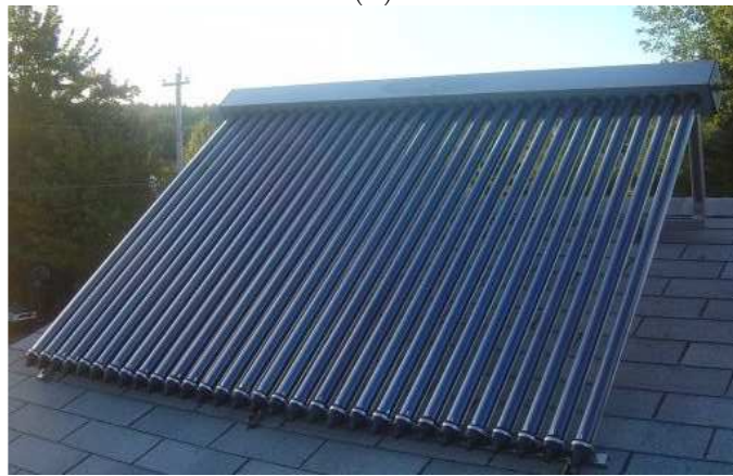
Figure 1.3: (a) Close-up view of an evacuated-tube collector. (b) A typical evacuated-tube collector system for residential water heating. Courtesy of Beyond Oil Solar.
